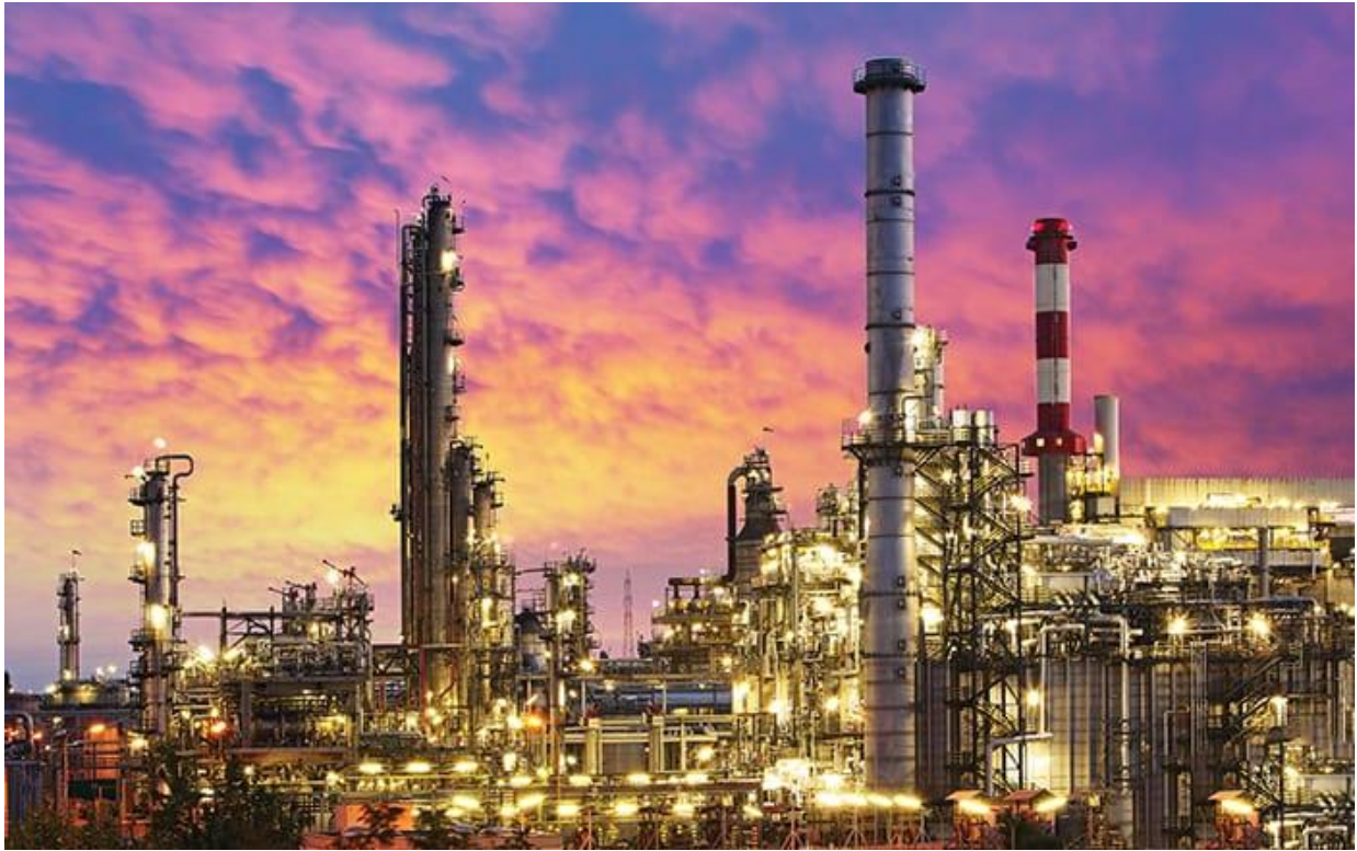
Figure 3. Simulation used throughout the entire plant asset lifecycle improves safety and other pillars of operational excellence
